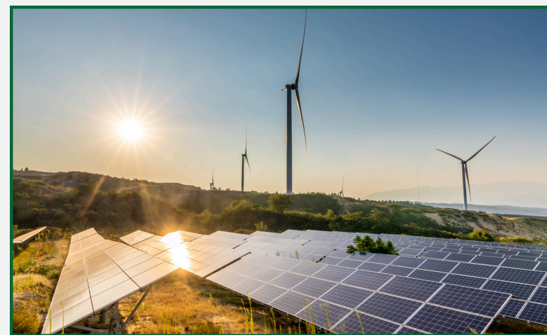
Wind Power Energy
