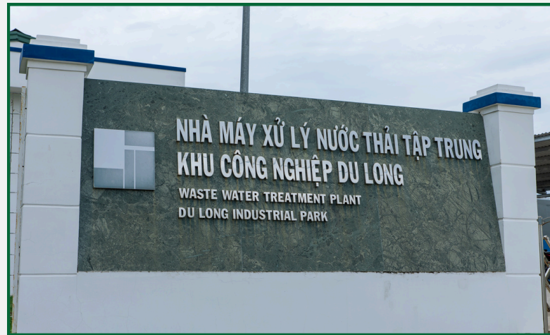
Water Treatment Plant with SBR Technology
