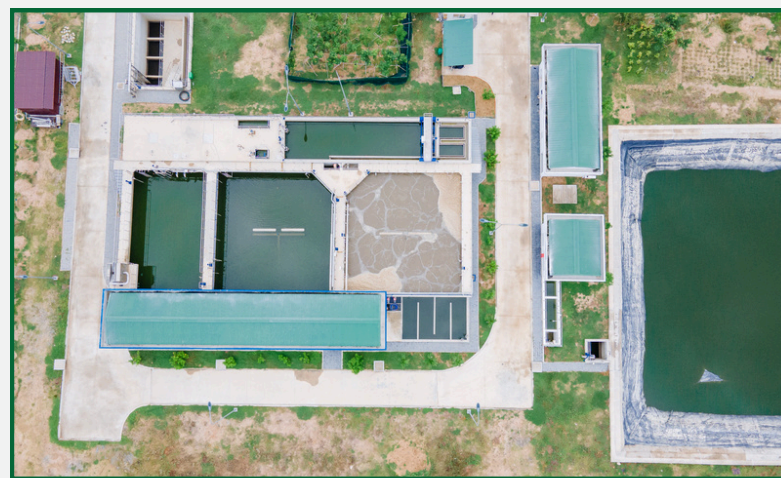
Waste Water Treatment Facility
