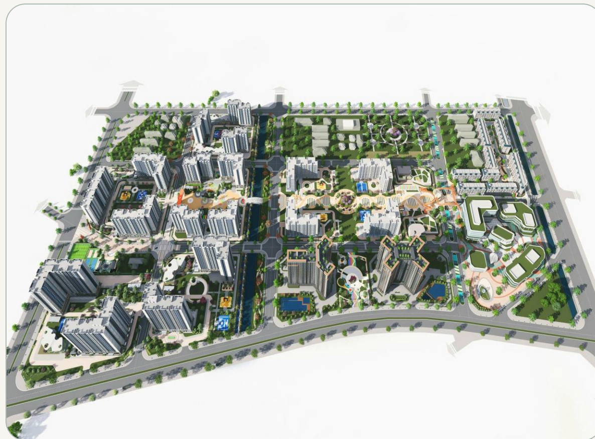
Tien Duong Park City social-housing project under development, with total investment of approximately VND 9.3 trillion in Phuc Thinh Commune, Hanoi
