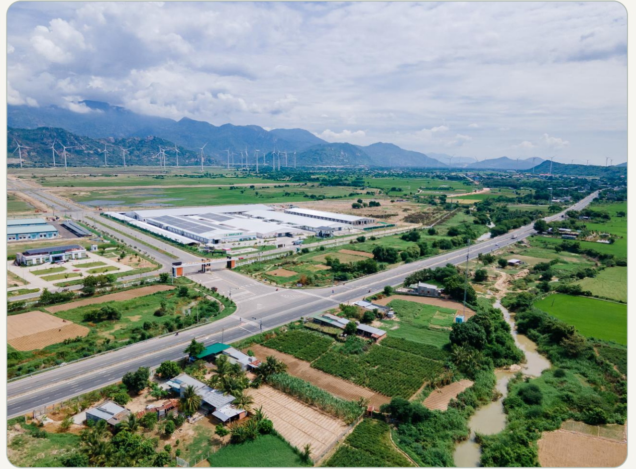
Industrial Park overview at National Highway 1A, Thuan Bac Commune, Khanh Hoa Province
