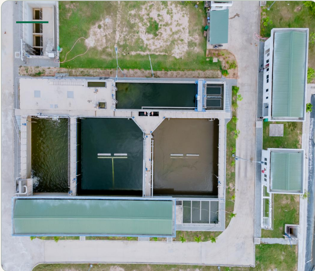
Aerial image of wastewater-treatment plant – Module 01
